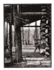
This detail shows the use of lock-notches at corners, and treatment of the butts
