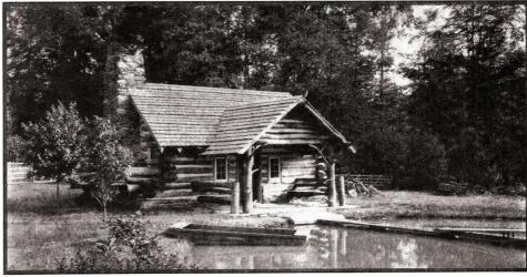
This log cabin has many interesting features. The hooded porch, sturdy chimney, walls pointed with mortar, and double row of shingles in every third course, are all in accord with the rugged scale of log construction
